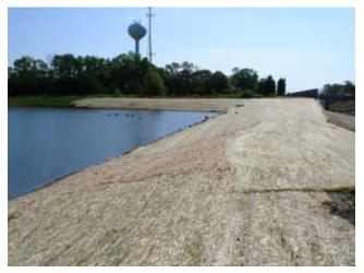
Erosion control blanket stabilizes pond slopes.
