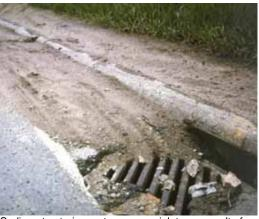
Sediment entering a storm sewer inlet as a result of construction related erosion.
